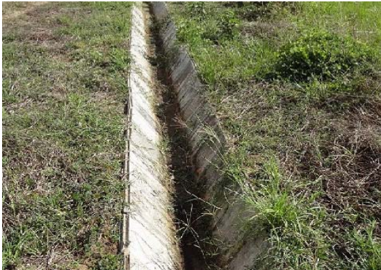
Grade -1: No serious deterioration No remarkable deterioration. Keep periodical monitoring.
