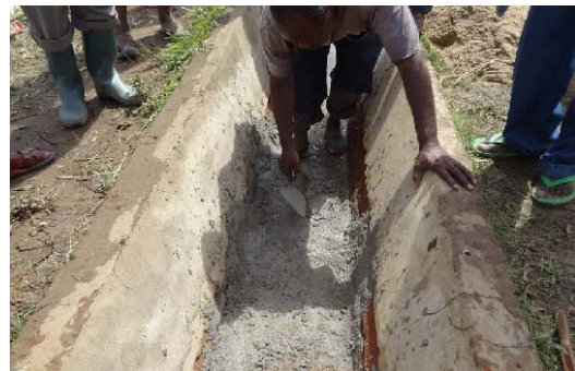
Filling blind mortar in hollow and removed parts
