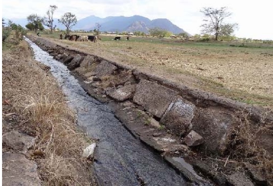
Grade- 4 : Collapse of slabs Long section damage, large scale rehabilitation needed.
