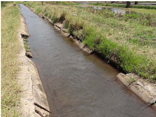
3 rd stage washout damage
