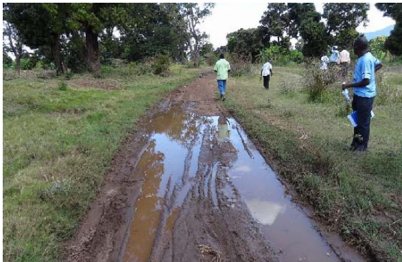
Grade- 2 ; Shallow wheel rut Shallow wheel rut/ muddy surface. But possible to pass with slow speed.
