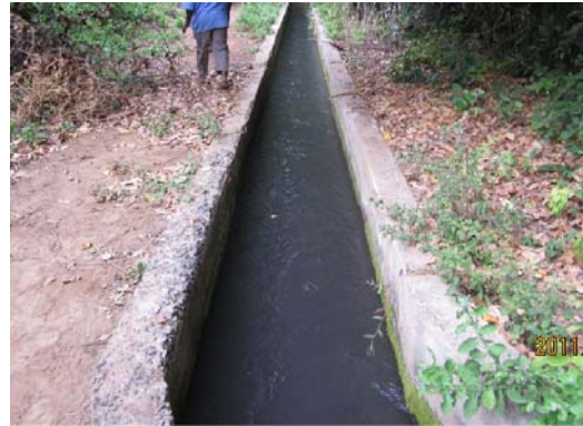
Grade -1or2 : Segregation of surface concrete Segregation of cover surface can be identified. But little problem for normal operation and function of facilities. Keep periodical monitoring.
