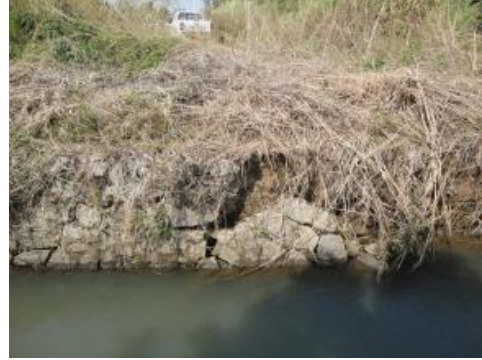
Grade-3or4 : Collapse of stone wall In case of partial section damage, then Grade3. In case of long section damage, then Grade 4
