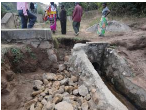
Grade-4: Washout of division point Normal operation impossible and unusable. Rehabilitation is needed
