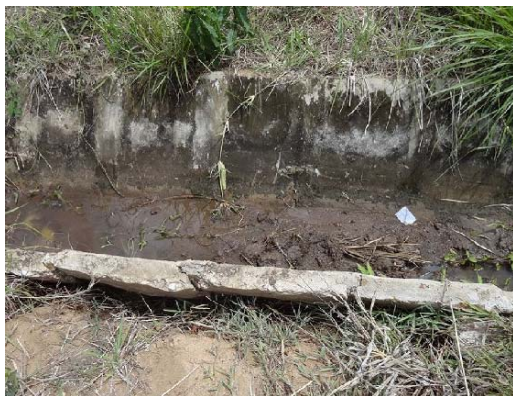
Grade-2: Hollow behind slabs Filling of hollow behind slab is needed to prevent development of damages.
