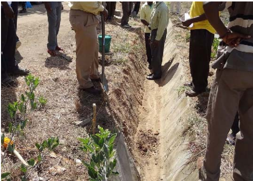
Removing deformed slab and clear dirt and weeds
