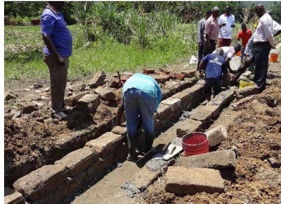
Installation of cement blocks
