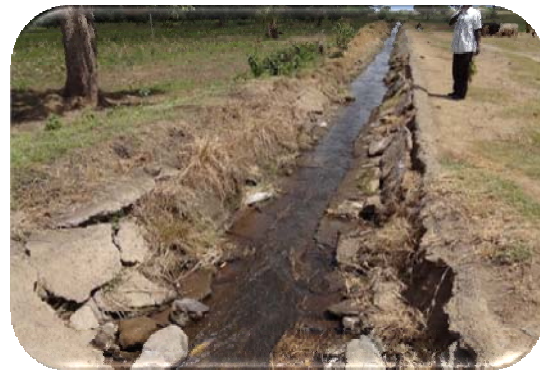
Example of canals that need large scale rehabilitation, As No Preventive repair work was conducted
