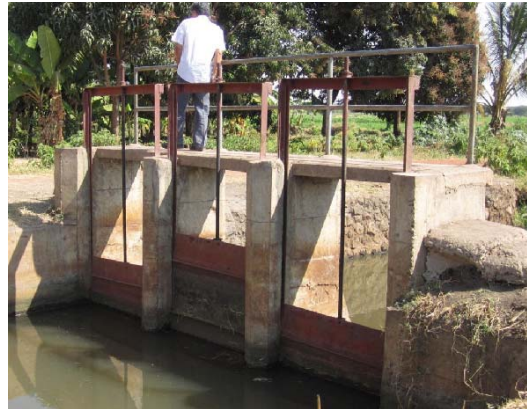
Grade- 1or2 ; Small rust of gate ; Normal operation possible. Keep periodical maintenance works
