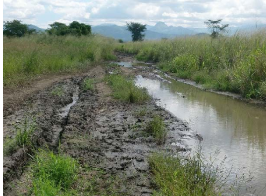
Grade- 4 ; Muddy and drainage problem Impossible to pass. Large scale rehabilitation necessary
