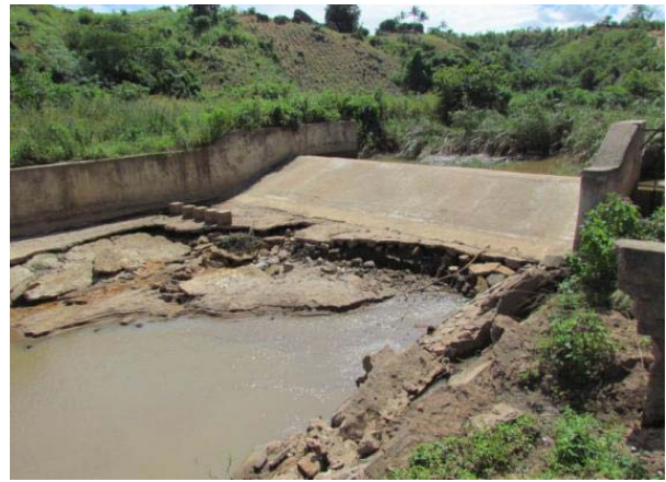
Grade- 4 ; Damaged head work Large scale rehabilitation is needed.
