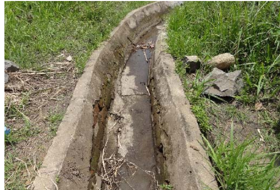
Grade-2: Abrasion wear of plastering cover Repair of plastering is needed to stop development of damages.
