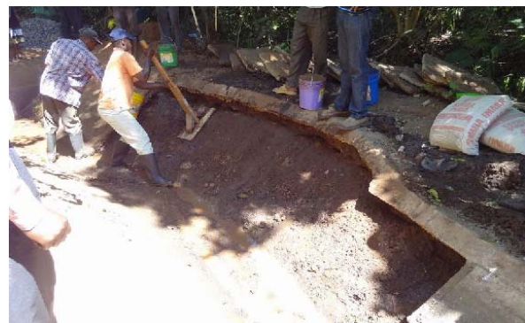
Remove of deteriorated slabs and filling soil.
