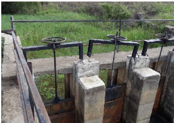
Grade- 4 ; Broken metal frame Frame of gate is completely broken Renewal of gate is needed.
