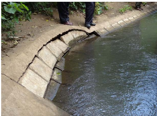
Deterioration Before repair work
