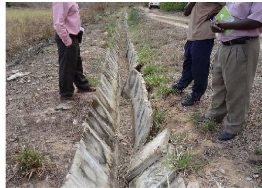
Grade-3 : Collapse of slabs Partial section damage and Partial section repair works can be applied.
