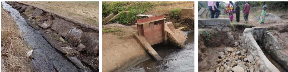
Images of deteriorated irrigation facilities
