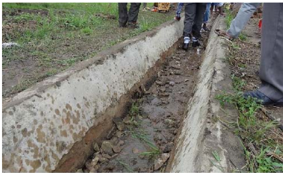
Removing deteriorated parts with chiseling and hummer
