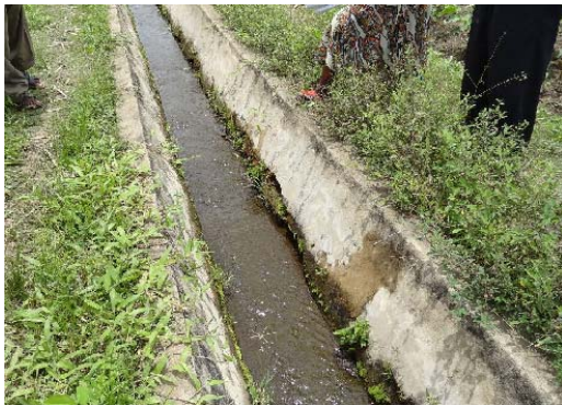
Grade-3: Loss of corner plastering cover Deterioration of corner part and leakage. Repair with new hunching concrete is needed.
