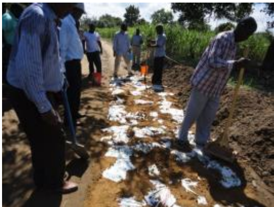
Filling spaces with murrum and compaction. (Two layers sandbags)
