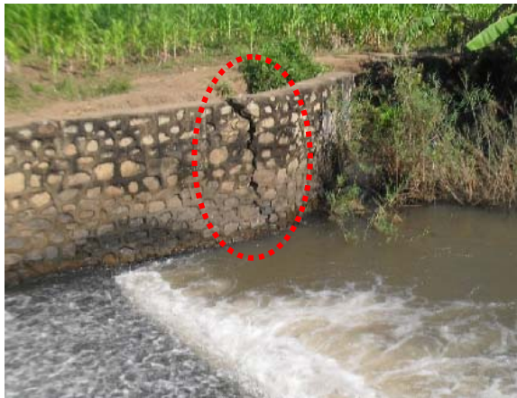
Grade-:2or3 : Crack on wall Repair of cracks is needed to prevent development of damages.
