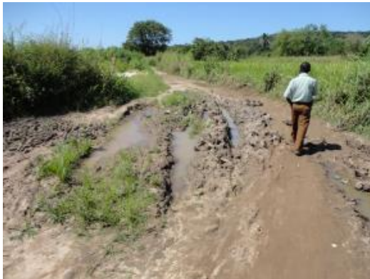
Grade- 3 ; Deep wheel rut/ muddy surface Difficult to pass for Deep wheel rut/ muddy surface. Damaged section needs repairing.
