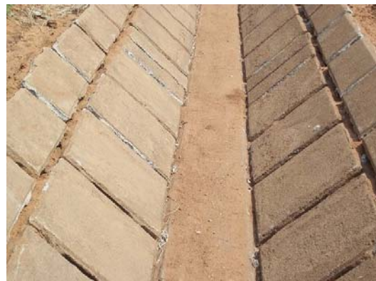
Grade-2: Loss of joint mortar Repair of joint mortar is needed to prevent development of damages.
