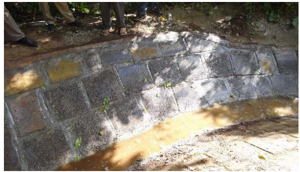
After repair works
