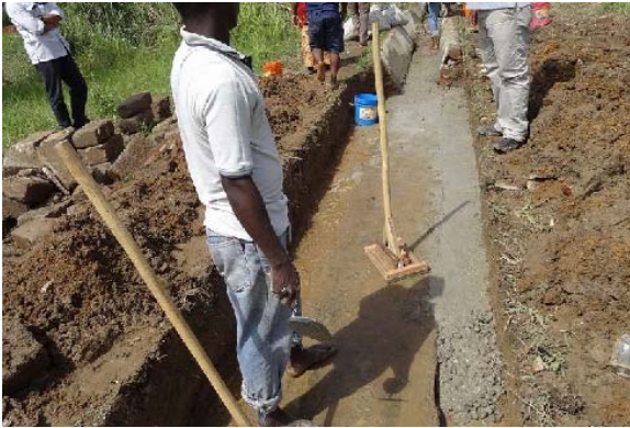
Excavation and casting base concrete
