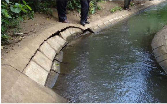
Grade-3: Deform of slabs Partial section damage and Partial section repair works can be applied.
