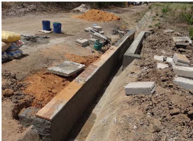
Example of partial repair with Cement Block
