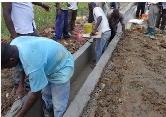
Plastering surface of cement blocks.
