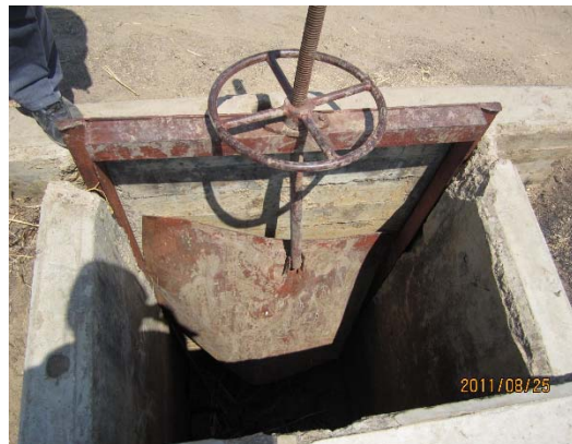
Grade- 4 ;Deform of gate plate Plate of gate is completely bent Renewal of gate is needed.
