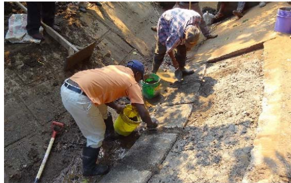
Re-installation of slabs (reused slabs)
