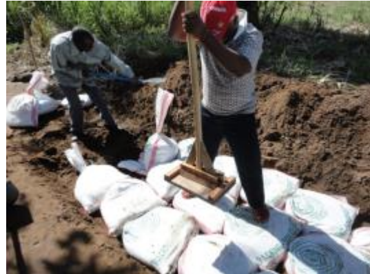
Installation of sandbags and compaction. (1 st layer)
