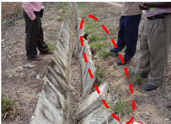
Runoff water penetrates behind of slab and washed out
