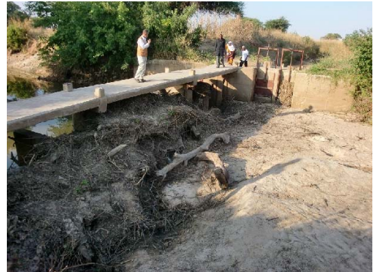
Grade-3 ; Heavy deposits around intake Normal operation is impossible. Cleaning is needed as soon as possible.
