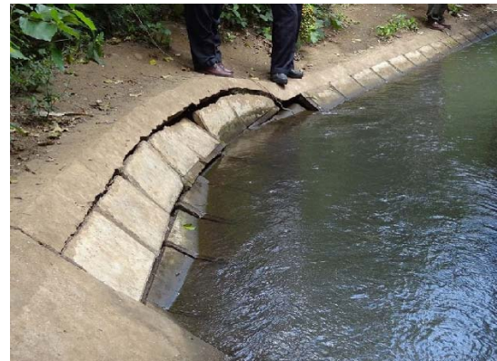
2 nd stage washout damage
