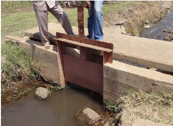
Grade-1or2 ; Small rust of gate Normal operation possible. Keep periodical maintenance works
