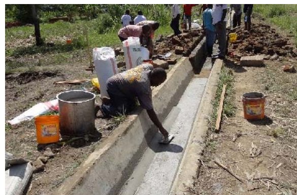
Casting haunch mortar and finishing surface with trowel
