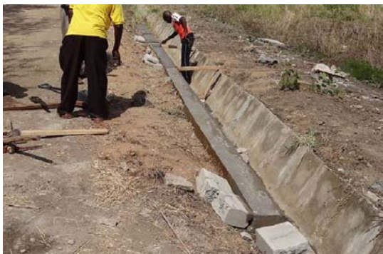
Casting capping concrete
