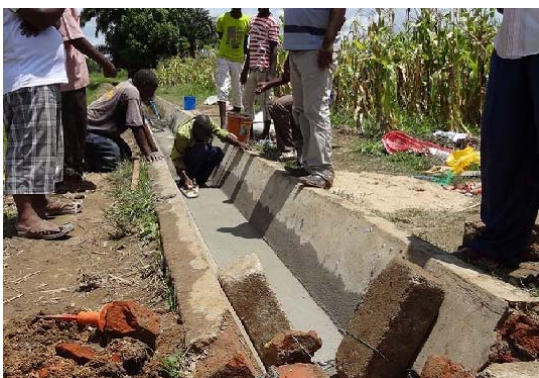
Casting base mortar (20mm) and finishing surface
