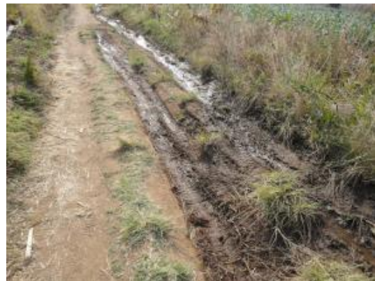
Grade- 2or3 ; Deep wheel rut Getting difficult to pass for Deep wheel rut/ muddy surface. Need diversion for passing
