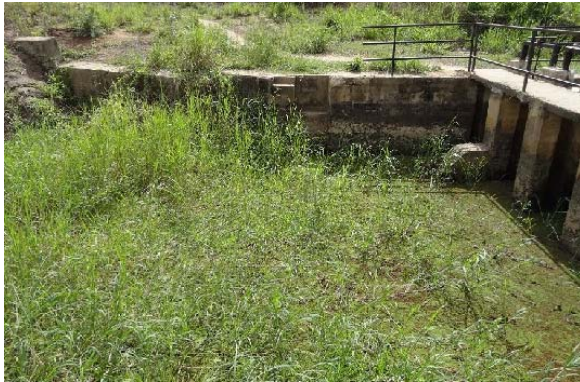
Grade- 2 ; Thickly weeded intake Normal operation is possible. But weeds may disturb intaking of water in near future. Cleaning is needed.
