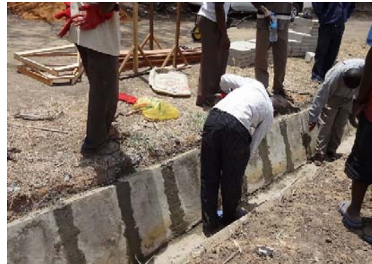
Re-installation of removed slabs
