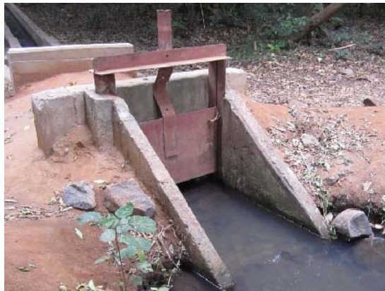
Grade- 3 : Deform of gate Normal operation difficult. Repair of handle is needed
