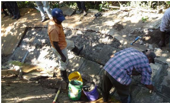
Re-installation of slabs (reused slabs)
