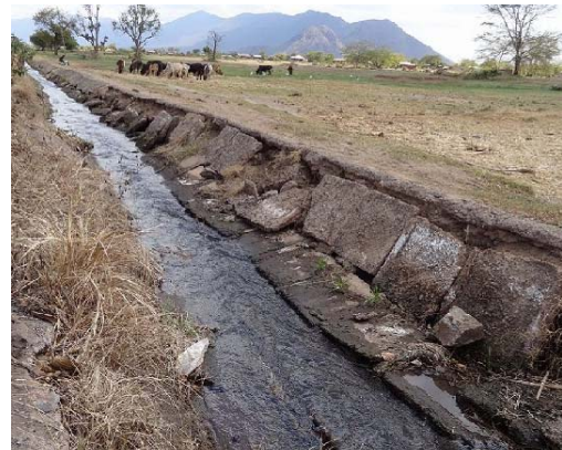
4 th stage washout damage
