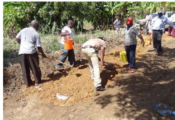
Put covering murrum soil (5cm deep) on sandbags and give Compaction, and make 5cm deep coverage layer
