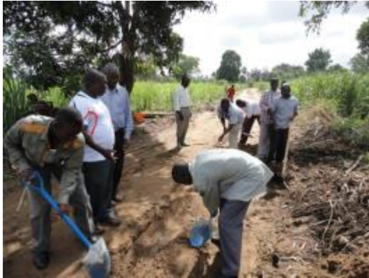
Excavation of targeted area. (25cm deep.)
