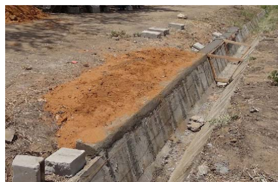
Backfilling and slope the surface for drainage.
