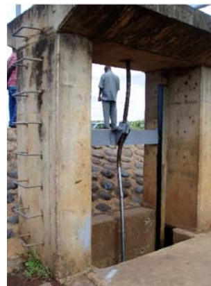
Grade- 3 : Deform of spindle Normal operation difficult. Repair of spindle is needed
