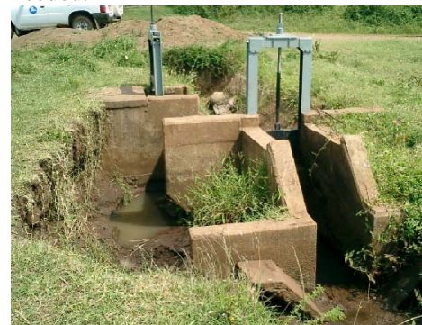
Grade- 4: Washout of division point Normal operation impossible and unusable. Rehabilitation is needed
