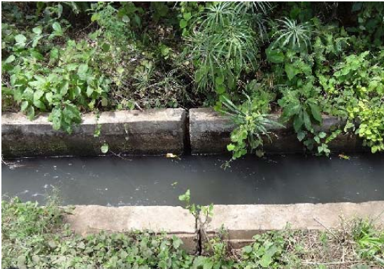
Grade-2: Gap of expansion joints Repair of joint is needed to stop leakage and wash out of soils.
