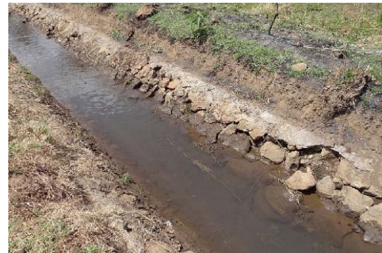
Grade-4 :Collapse of stone wall Long section damage, large scale rehabilitation needed.
