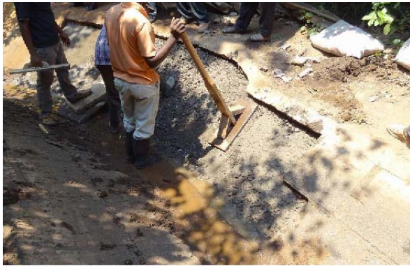
Casting backfilling concrete
