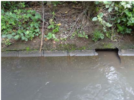
1 st stage washout damage
